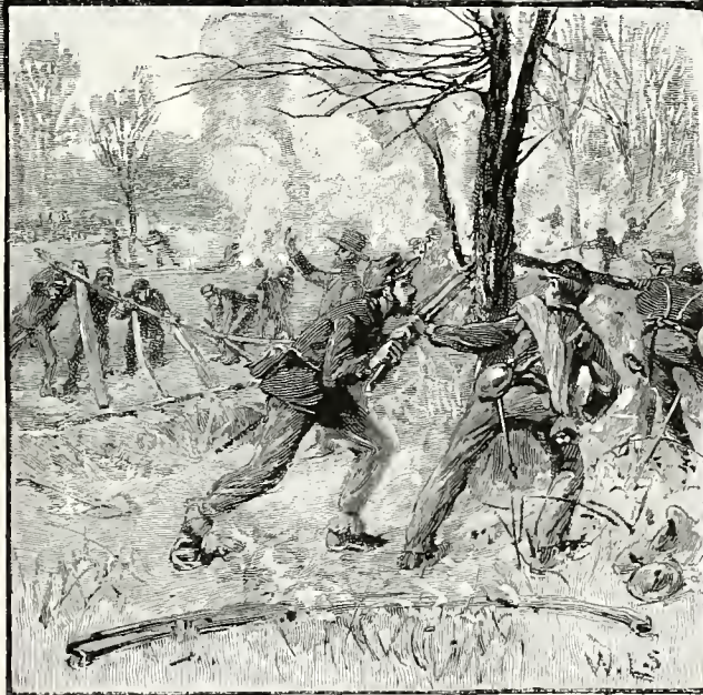
DESTROYING A RAILROAD.
